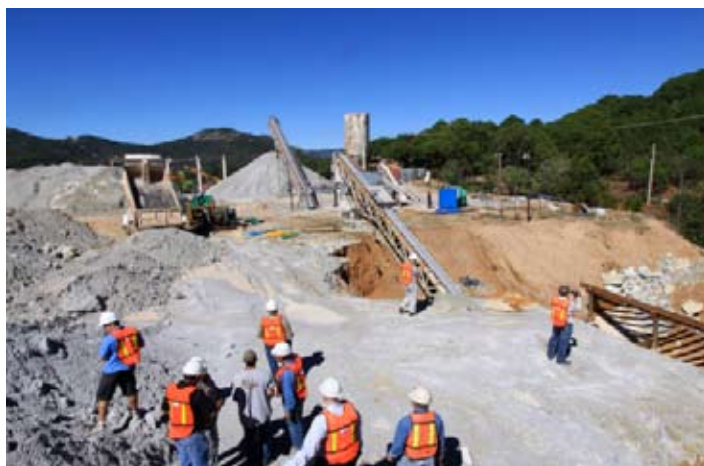
Oct 09 - gold ore being unloaded into the grinding circuit as analysts watch
